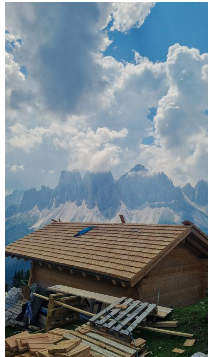
The cold shell for the new hut.
